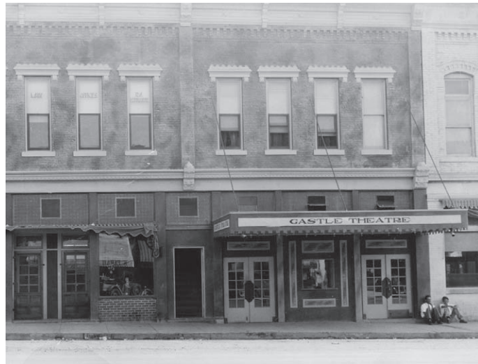
In the 1930s Ora & Shorty Cleveland built and operated the Castle Theatre. In April of 1939 the west wall of the Castle collapsed. It was theorized that the water soaked ground and the excavation of the building next door caused the collapse of the Castle Theatre. (Photo Courtesy of Anna Miller Museum)
