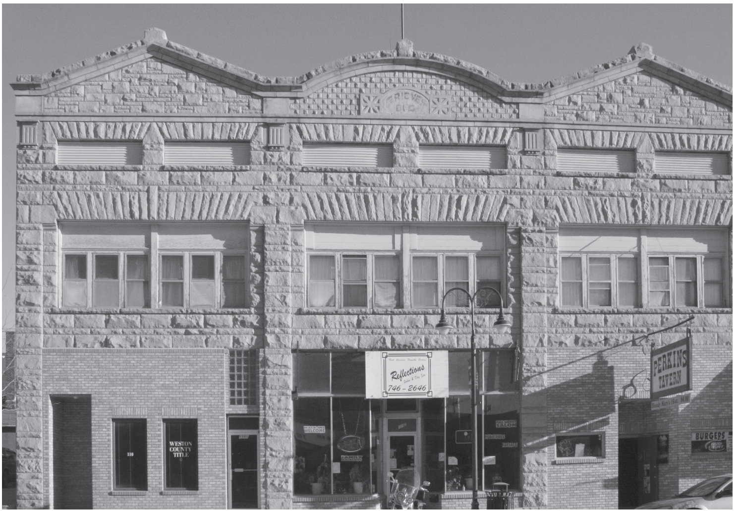
The Nichols building is still standing after a hundred years. Photo taken in 2012.
