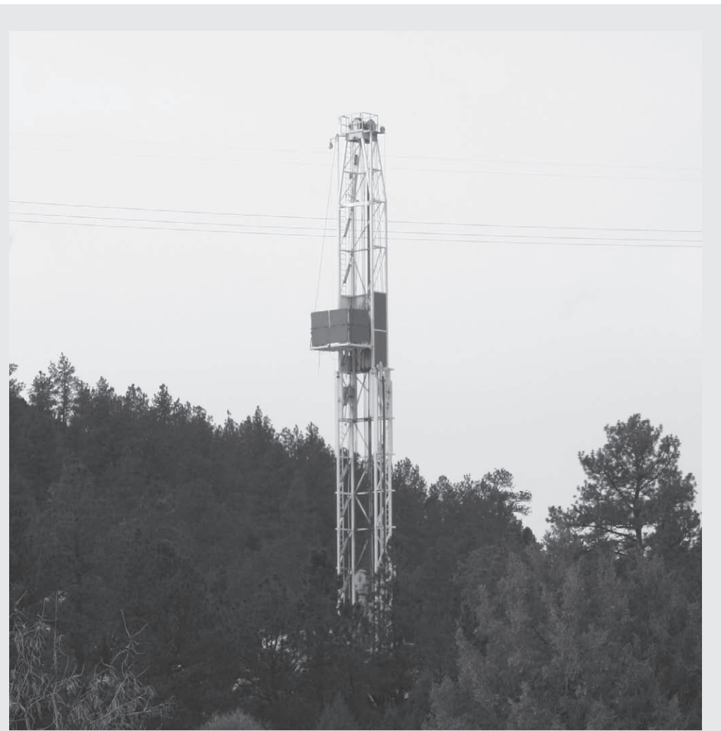
A drilling rig rises above the tree line near the Newcastle City Shop, and should reach the Madison Formation in about a month. (Alexis Barker/NLJ)
