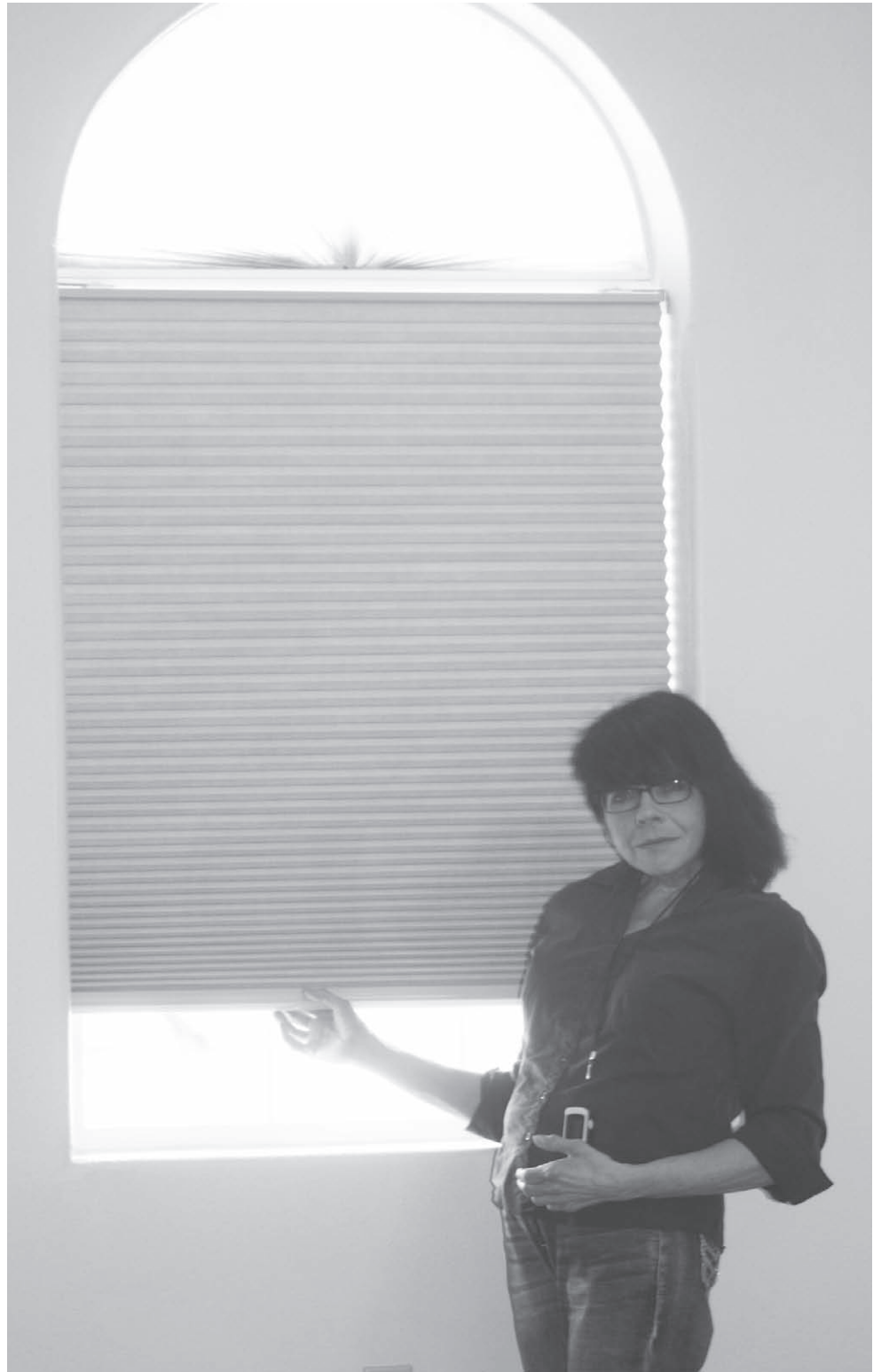
Laurie Martin demonstrates some of the window treatments she has recently installed for a customer in Weston County. (Pam Penfield/NLJ)
