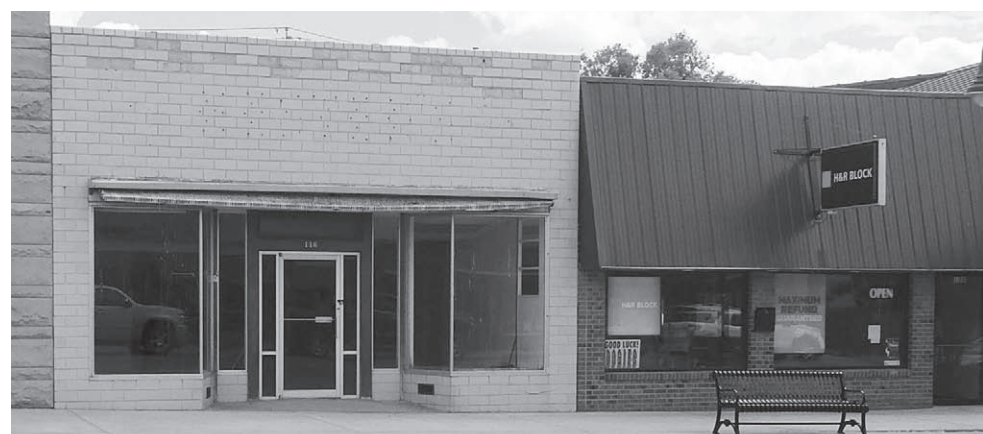
The appearance of both the business front and the sidewalk was improved substantially when the old wooden awning was taken down. (Submitted Photos)
